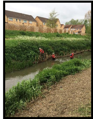
A faggot; floating into position; stamping down;
