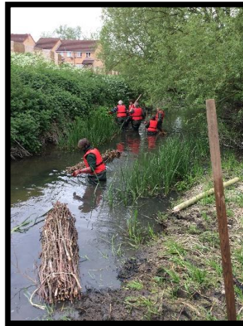
A faggot; floating into position; stamping down;
